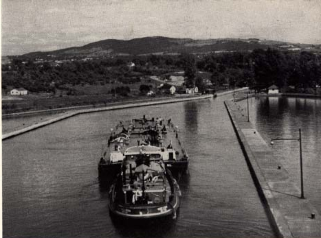
DOWN THE FLIGHT —The tug Marie S. Moran with Texaco's barge No. 397, entering Lock No. 4, the central one of five which drop the New York State Barge Canal 169 feet around the Great Falls of the Mohawk River to the Troy level of the Hudson River. The Troy level (above the government lock) is approximately 15 feet above the Hudson at sea level. This is a typically attractive scene along the great Empire State waterway, seasonal assignment to which most veteran canalers emphatically prefer to the hurly-burly and frequent discomfort of winter work in and around New York Harbor when the canal is frozen over.
