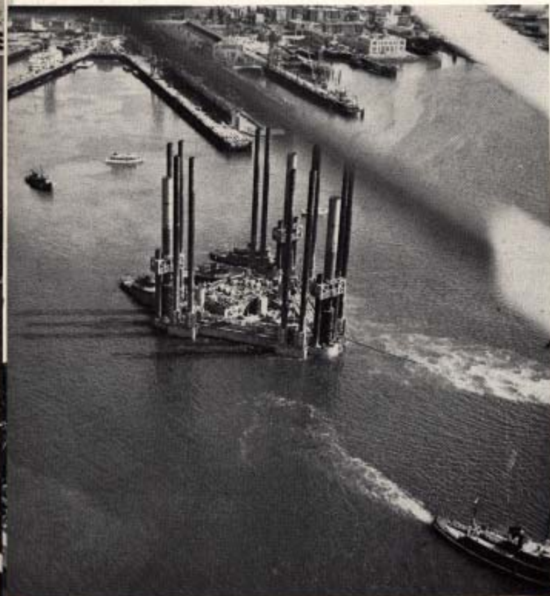
With two local tugs assisting Moran's ocean tugs, tower moves slowly into main ship channel
