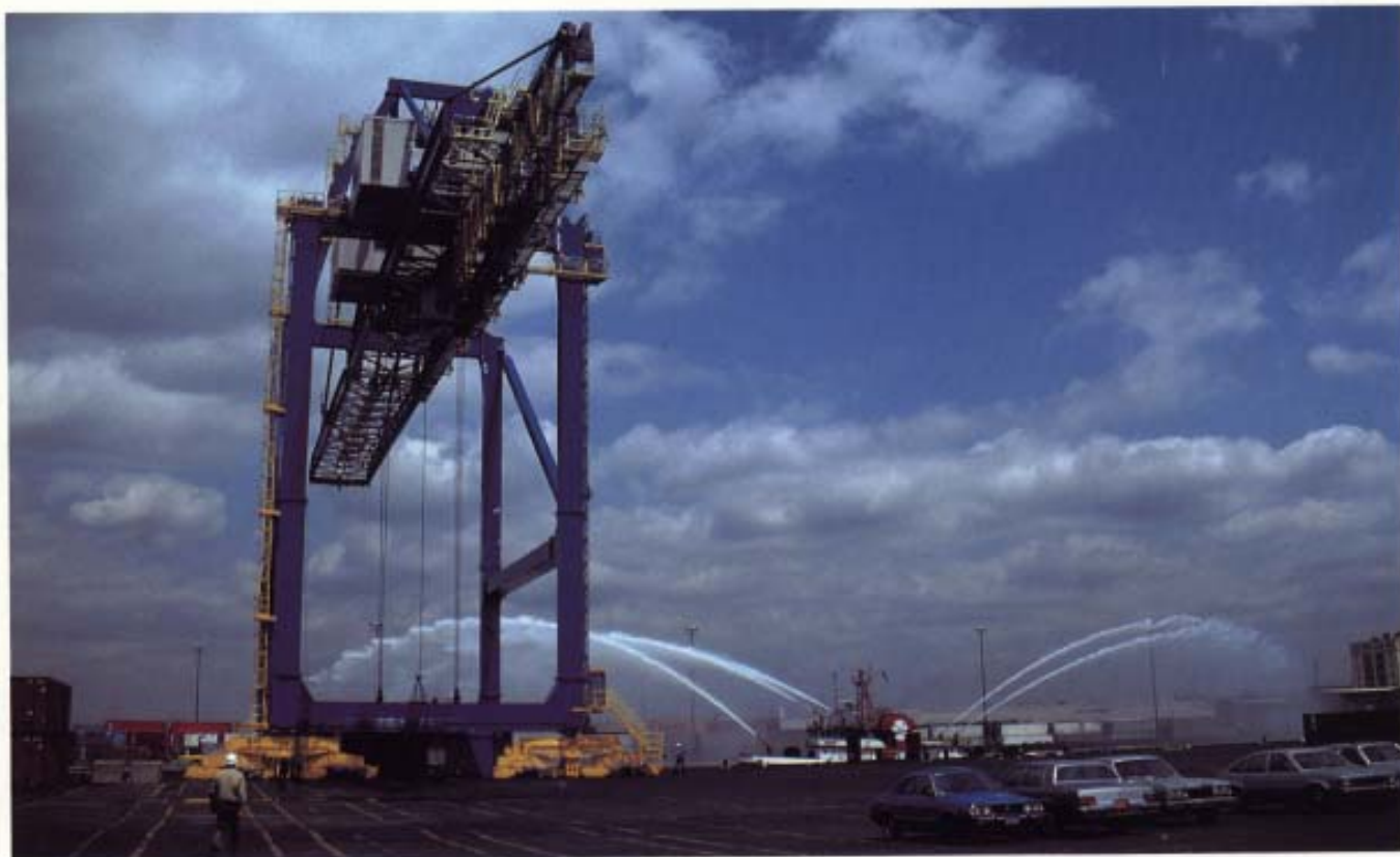
The new $3 million container crane at the South Brooklyn Marine Terminal, Brooklyn, N.Y. receives a fireboat salute at the dedication this past May.
