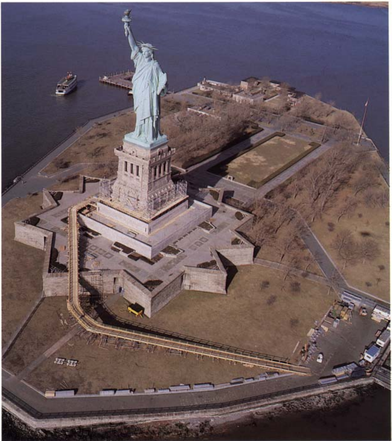
THE STATUE OF LIBERTY —The stage and the staging for the careful restoration and preservation of the Statue of Liberty—and for Miss Liberty's upcoming Centennial Celebration in the Port of New York July 4, 1986—is being set in this TOW LINE photograph of February 22, 1984. The lengthy, inclined ramp to the base of the statue is in place—already carrying a stream of scaffolding which will eventually completely envelop the 152' tall Symbol of Freedom. Restoration materials are to be fed internally to the statue through an access port cut in Liberty's left sandal at the heel. The initial staging is visible in the photograph, each day growing higher. This gift of the people of France to the people of the United States to commemorate the alliance of France and the United States in our War of Independence was originally presented to the American Minister to France (Levi P. Morton) in Paris on the 4th of July 1884. In New York on the 28th of October 1886, President Grover Cleveland dedicated the completed Statue of Liberty on her pedestal on Bedloe's Island. In 1956, the name of the island was changed by a Resolution of Congress to Liberty Island.
