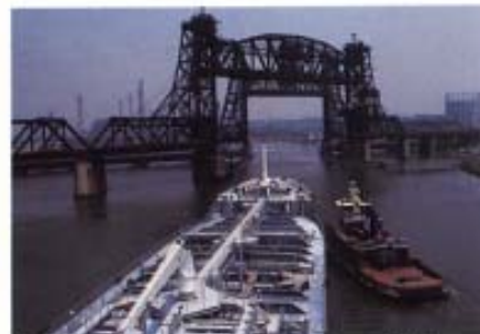
Rt. 10 Hiway & two Penn. Railroad bridges require expert navigation.
