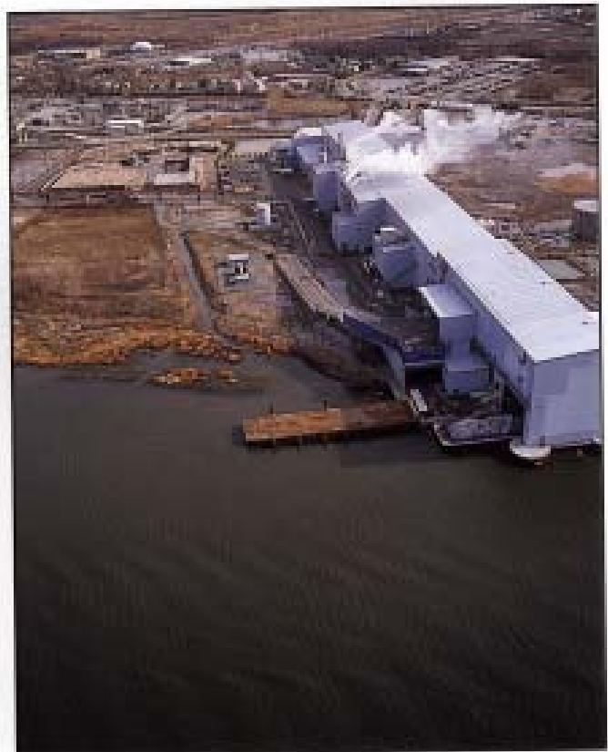
An aerial view of the new 1,300-foot long Visy Recycling plant, located in the Travis section of Staten Island, N.Y., on the Arthur Kill Waterway.
