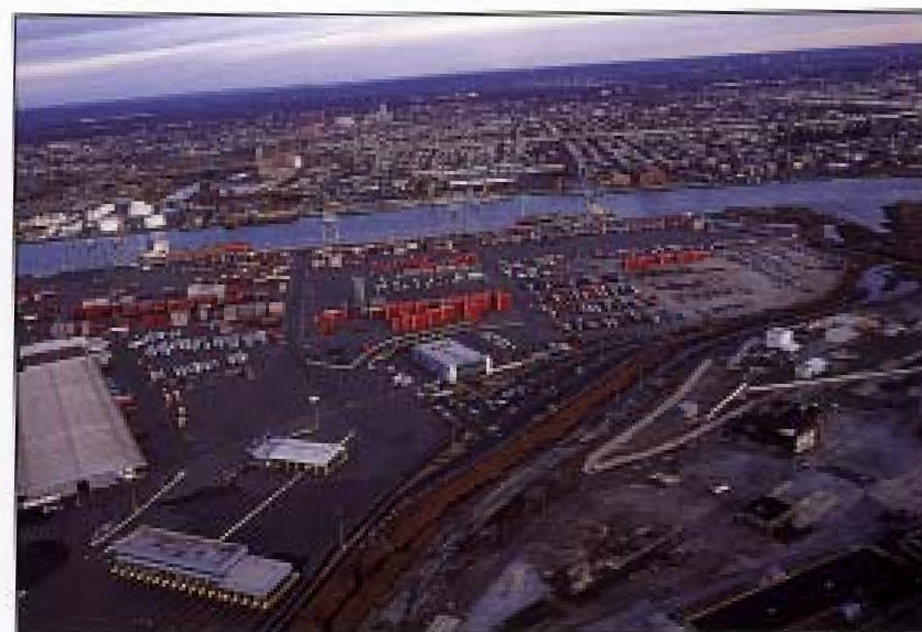
The Howland Hook Container Terminal, Staten Island, looking toward the Arthur Kill Waterway.
