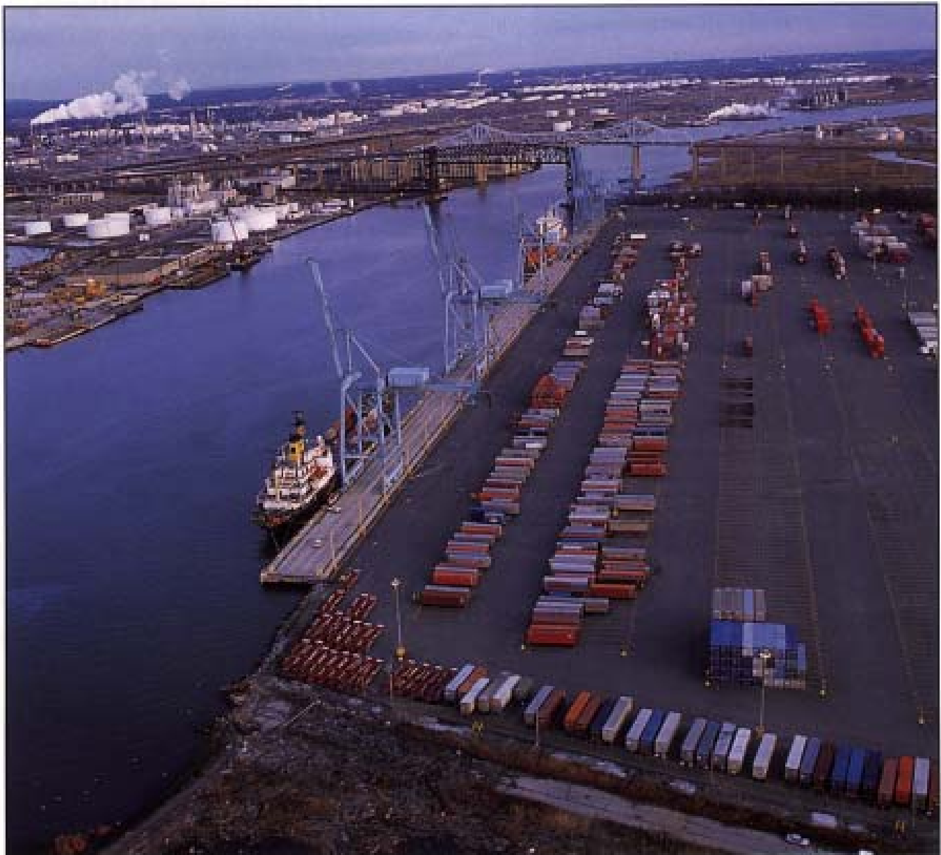
The newly reopened Howland Hook Container Terminal has the capacity to handle 425,000 containers annually.
