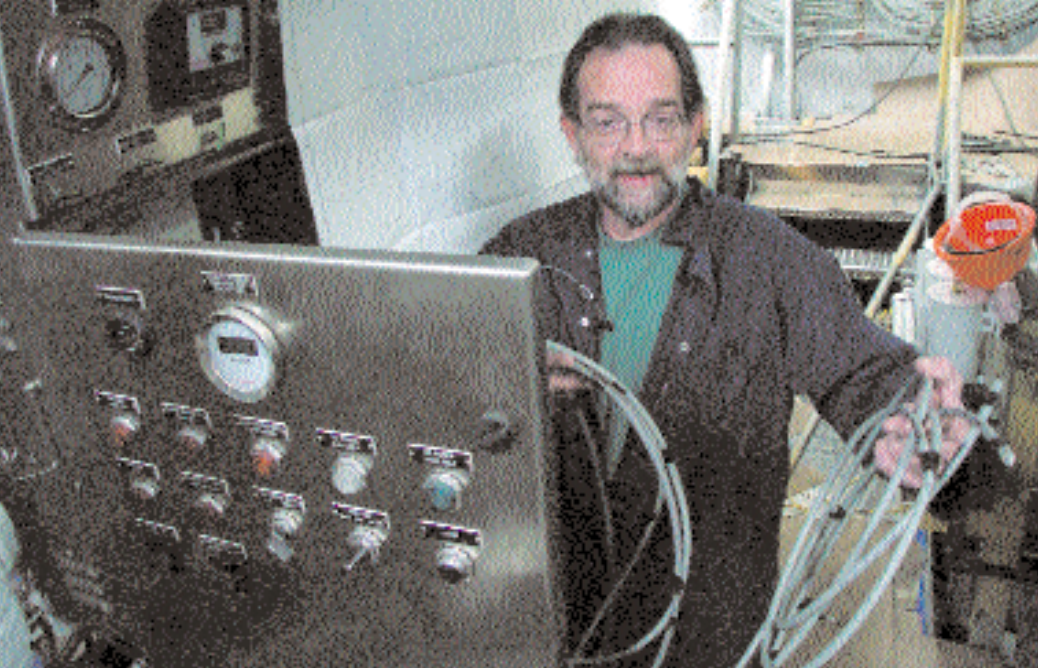
Eddie Sanders, port engineer at MORAN's Norfolk division, has been on hand for final fitting out of many of the company's new tugs in Maine. At left, he explains wiring being installed in a control panel aboard the Edward J. Moran . Below, Dave Missroon, captain, left, and Brian Miller, mate, attach the bitter end of ship assist hawser on the tug's Markey bow winch. Below left is a drive shaft with supporting bearing assembly equipped with electronic heat sensor. The drive shaft leads to a Rolls Royce z-drive unit.
