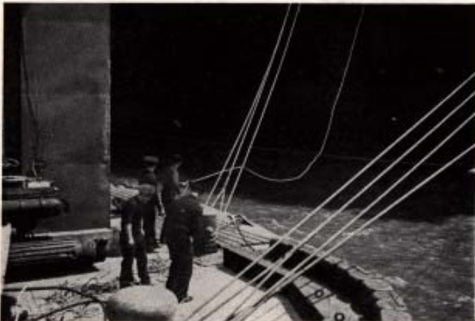
Mooring lines are made fast to dock bits.
