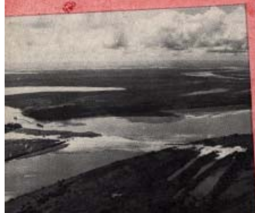
Aerial photo of Gahagan dredge working in typical Orinoco River delta country.
