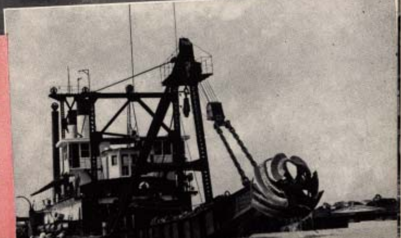
Right: Gahagan dredge PERU with dredging ladder elevated, showing formidable cutter-head.
