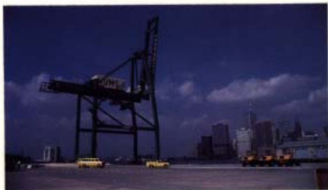
RED HOOK'S THIRD CRANE
